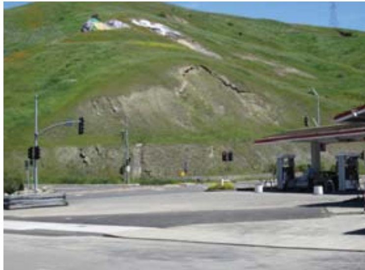
Rheem sinkhole repair complete
